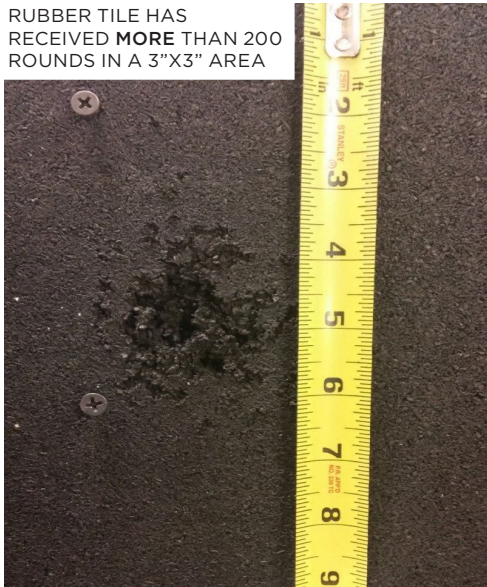
FIGURE 19. FRONT SIDE OF RUBBER PANEL NEEDS TO BE REPLACED
