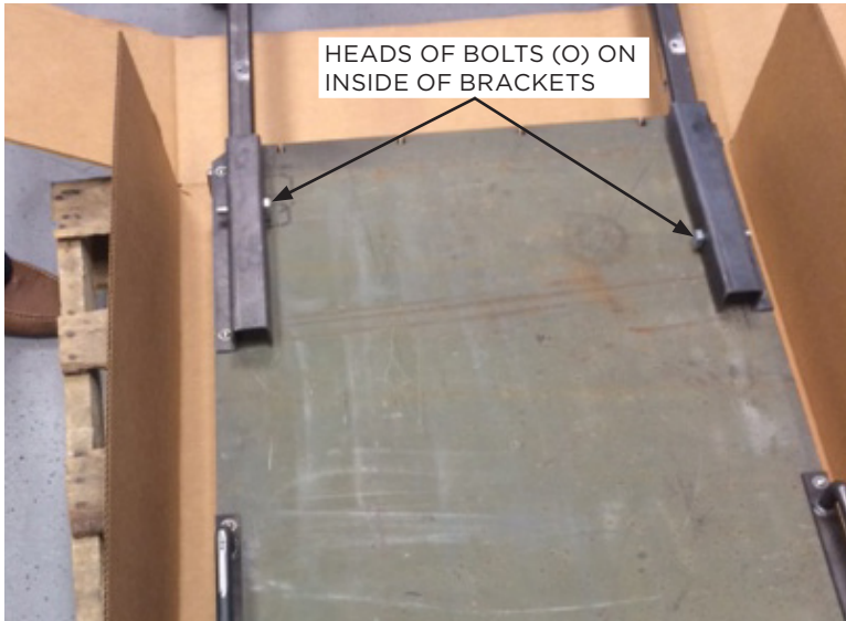
FIGURE 10. INSERT HEX BOLTS INTO BULLET TRAP PLATE BRACKETS
