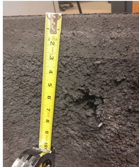
FIGURE 20. BACK SIDE OF RUBBER PANEL NEEDS TO BE REPLACED
